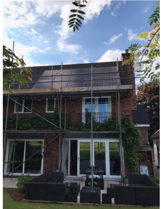
Image 2: Panel Installation in Progress
