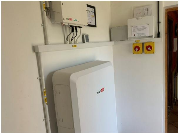
The whole of the Micro Generation system (the posh name for it!) has its own consumer unit, Fire service approved Isolators and is a fully compliant installation
