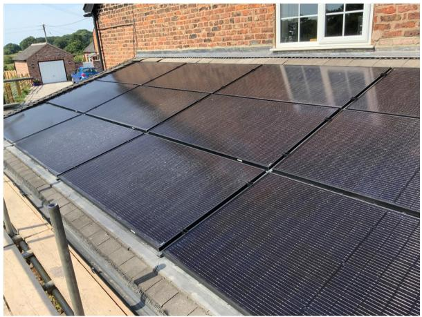
These feed into an Inverter/Control Unit and then the electricity the supply either powers appliances in the house, charges up a 10kWhour Battery or feeds into the
