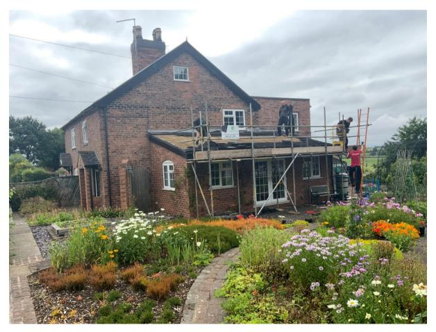
The low slope on the Music Room roof was also an issue. The most usual process of installing the panels is to fit support brackets that are screwed directly on to the rafters (bending round and through the tiling). This proved to be unworkable in this case as it would be hard to ensure that the panels were secure enough in windy weather; instead, we elected to remove the tiles and replace them with an integrated solar roof.
