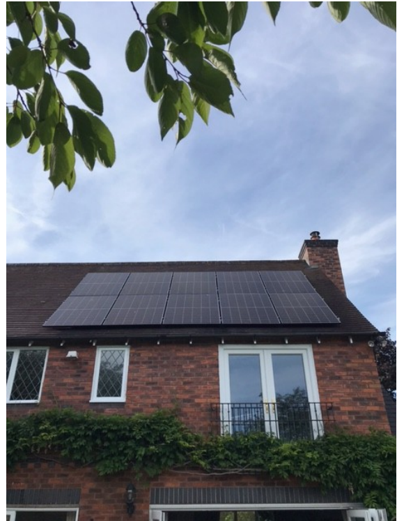
Image 6: Completed PV Panel Installation
