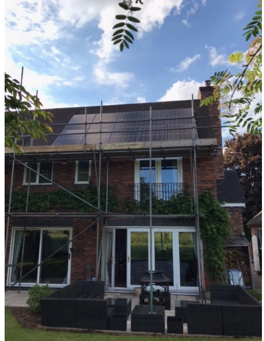
Image 2: Panel Installation in Progress
