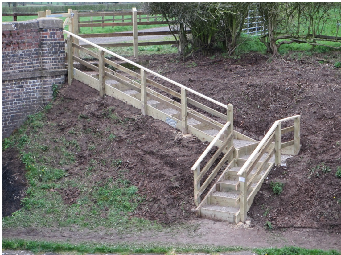
The end product – before the application of the stone top-dressing on the treads of the steps
